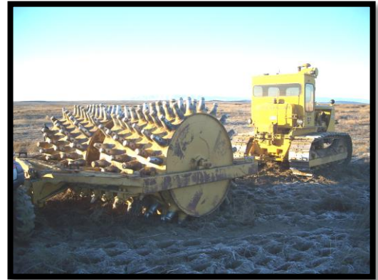
Figure 13. Sheeps-foot roller pulled by D-6 bulldozer
